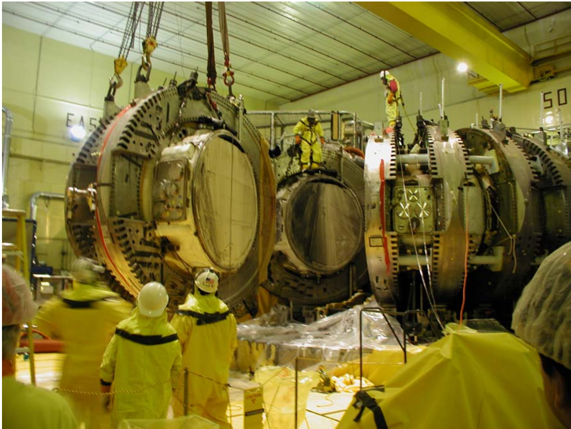
Figure 6 – Removal of First Segment
